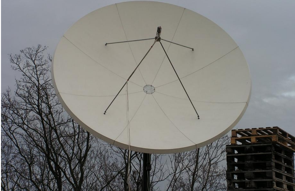
Satellite Express A4 at 14,0°W - Africa/Middle east beam in reception zone central Slovakia with PF 365 cm
